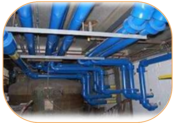
Piping Fabrication & Installation
