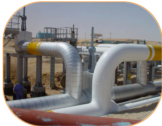
Gasco Buhasa Facilities Upgrading Project
